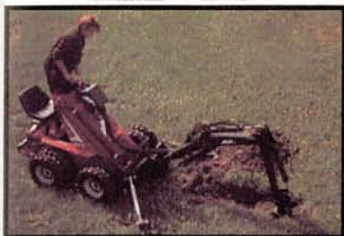
EXCAVATORS TO 2.7m
